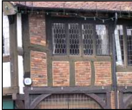
Close up of Angel Buildings
