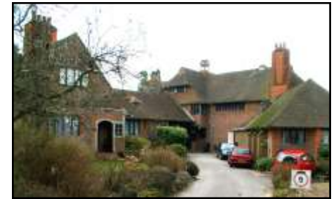
Weydown Road, Ballindune
