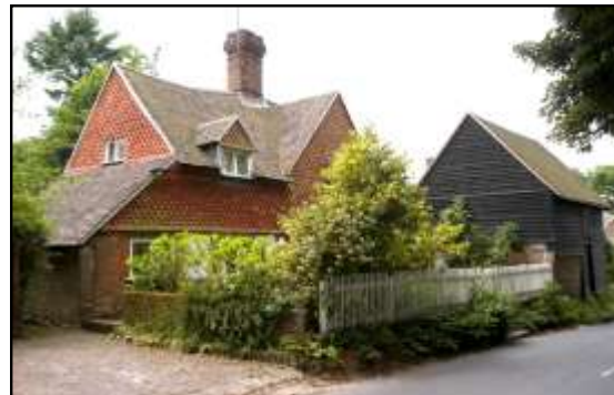
Little Barn, Church Lane
