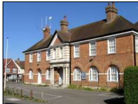
Former Police Station
